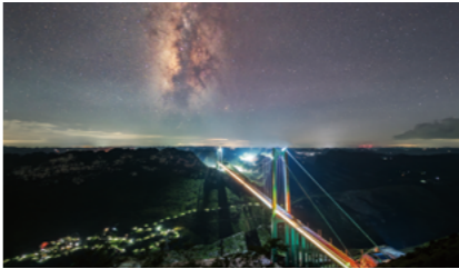
Huajiang Canyon Bridge, Anshun, Guizhou
