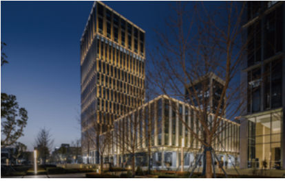
Hangzhou Haiwei Centre
