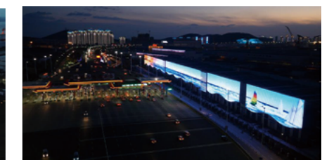
Qingdao West Bay New Area Motorway Entrance
