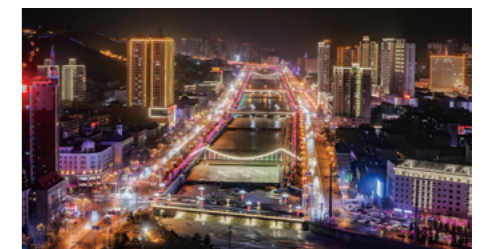
Lüliang City Lighting Project
