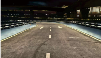
Xining Caojiabu Airport Motorway
