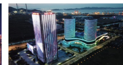
Zhoushan High-Tech Industrial Park
