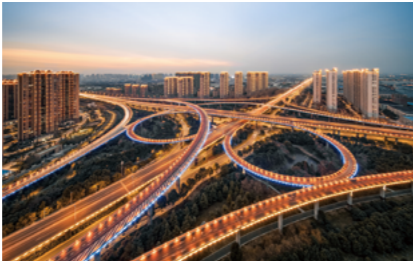
Changzhou Longcheng Elevated Road
